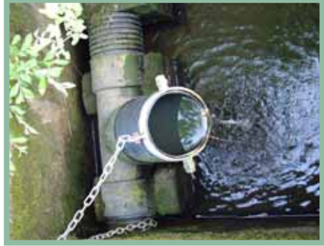
Figure 6: Simple water-level control mechanism.
