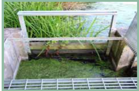
Figure 6: Simple water-level control mechanism.
