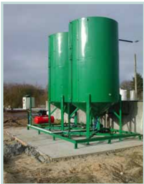
Figure 8 B: The sieve sludge sedimentation systems. The photo shows the fabricated equipment, each of the two tanks are 9\text{m}^3 in volume. The small box contains the control equipment including a PLC, relays and pneumatic control. A compressor is used to drive the pneumatic system that actuates the valves. The whole process is controlled by floating level sensors within the tanks which coordinate the emptying and filling of the tanks.
